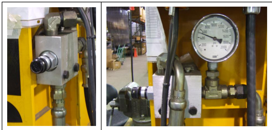
Fig. 7 – Pressure Control Valve (left) and Cylinder Pressure Gauge (right)
