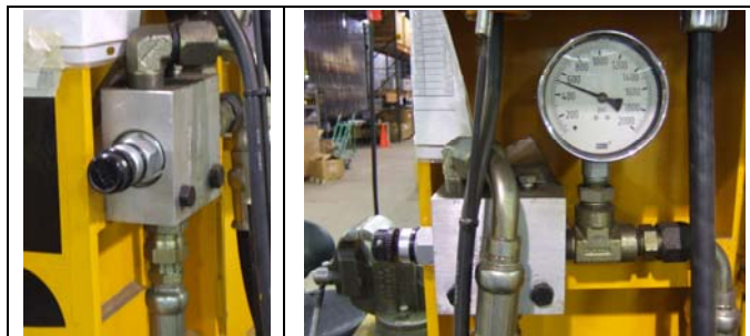
Figure 5 – Regulator and Cylinder Pressure Gauge
